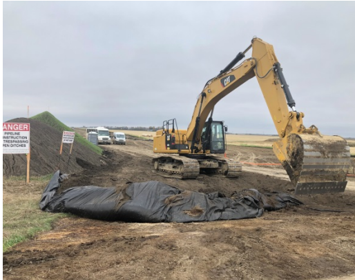
SF 3, photo facing west, excavator pulling geotech used for approach back onto ROW, getting rid of approach.
