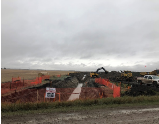
SF 25, photo facing east, one excavator widening out the sides of the trench.
