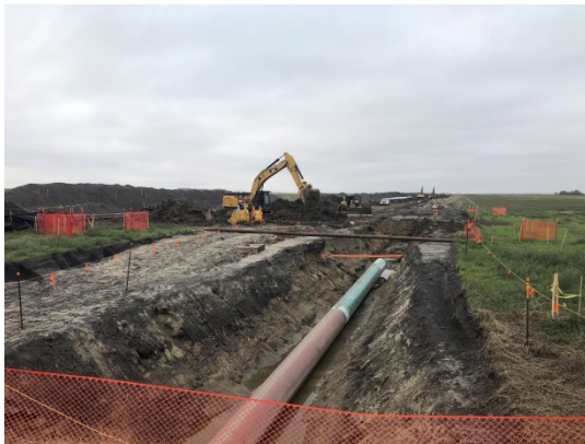
SF 5, photo facing west, excavator digging hole for where the valve will go on the ROW.
