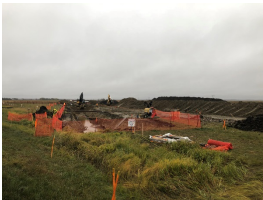
SF 22, photo facing south east, one excavator digging in the trench.
