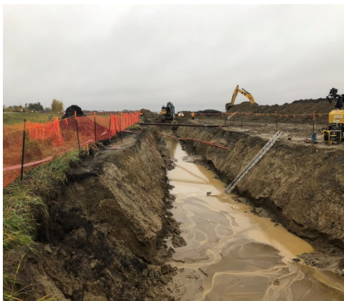
SF 22, photo facing south east, closer up photo of the trench full of water.
