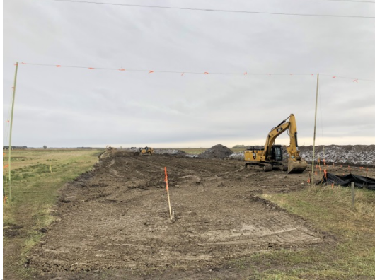
SF 3, photo facing east, one dozer pushing soil, one excavator parked.
