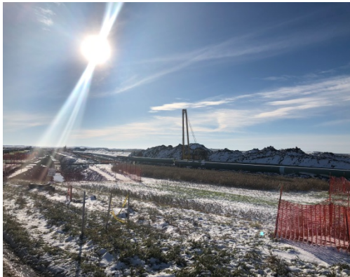
SF 24, photo facing south, crews heating the pipe.
