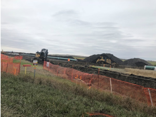
SF 24, photo facing south east, excavator digging hole for where pipe will come up from under the road, dozer pushing that soil to the side.
