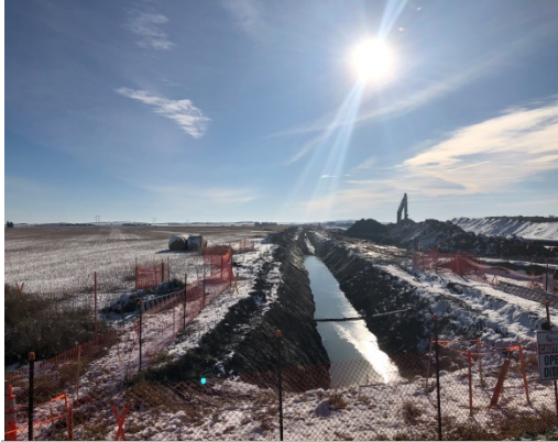
SF 25, photo facing west, excavator loading dirt into rock truck, rock truck dumping dirt into trench.
