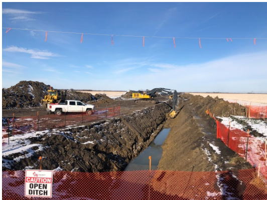
SF 25, photo facing west, excavator digging dirt out of trench.
