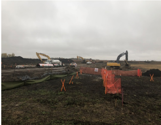
SF 20, photo facing west, one excavator digging in the trench, two more excavators moving dirt.
