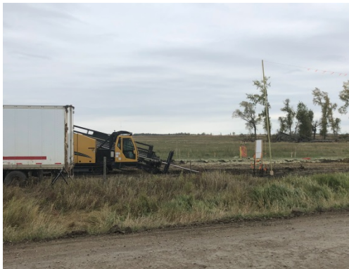
SF 22, photo facing north, machine drilling hole for pipe under the road.
