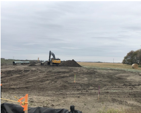
SF 26, photo facing north, excavator digging where trencher made the trench.
