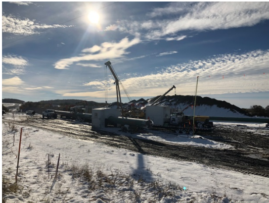
SF 35, coating crew coating the joints on the pipe. (south facing)
