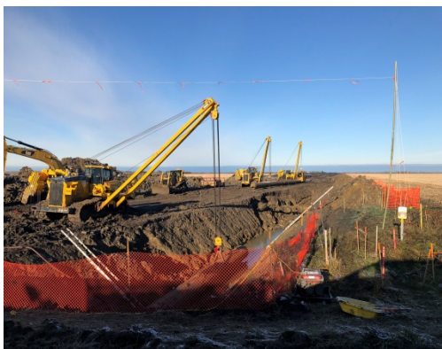
SF 25, photo facing west, lowering crew in, getting ready to lower in pipe.
