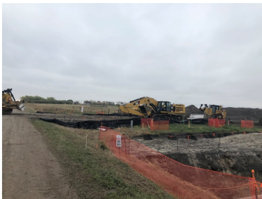
SF 5, photo facing south west, equipment crossing the road to be used on the west side.
