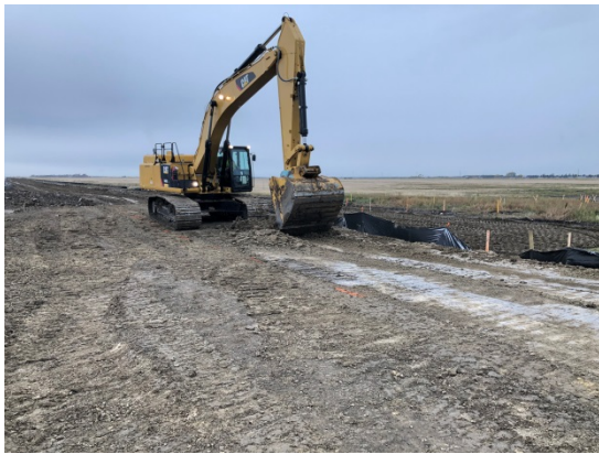
SF 4, photo facing west, excavator scraping rough mud off the approach.
