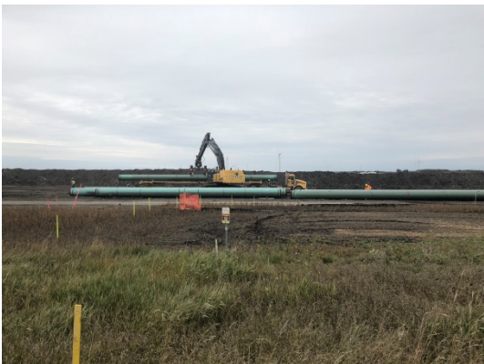
SF 48, photo facing west, excavator loading pipe onto semi-trailer.
