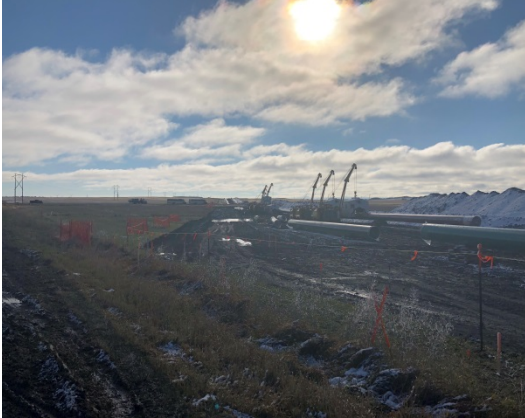
SF 43, photo facing south east, pipe gang working on the pipe, welding it together.
